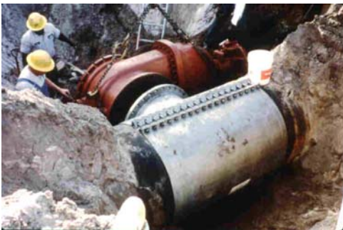
Tapping sleeve on distribution pipe
