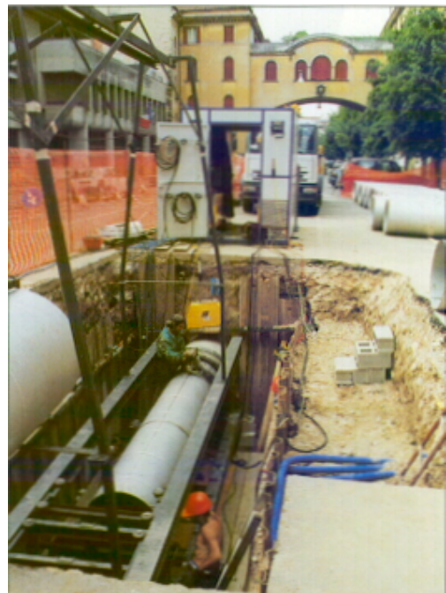
Trenchless relining of water main
