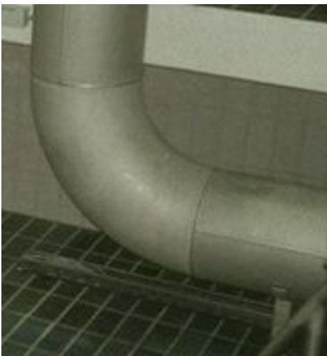
Good fabrication practice- Heat tint removed
